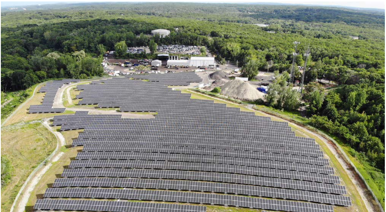
We invested in this 2.6 MW solar array in North Providence, Rhode Island, which is built on a former landfill site.
